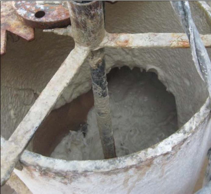
The slurry seen in this picture shows the type of coating that can occur in cyanide leach applications. The pH sensor is mounted on the end of the submersible dip tube in the center of the stilling well leading into an open vat. The recirculated leach solution is entering from the piping on the right.
